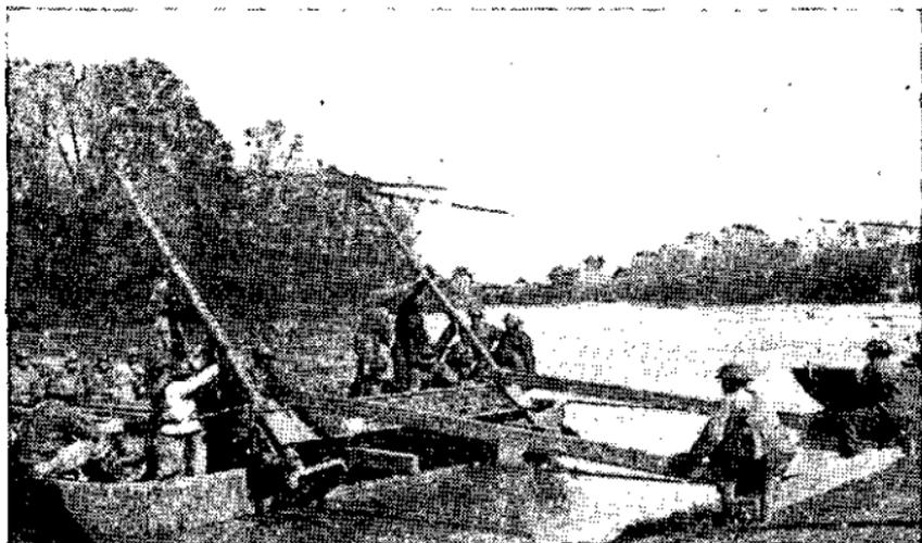
FIGURE 48.—Hinge sill raft being used for placing trestle.
