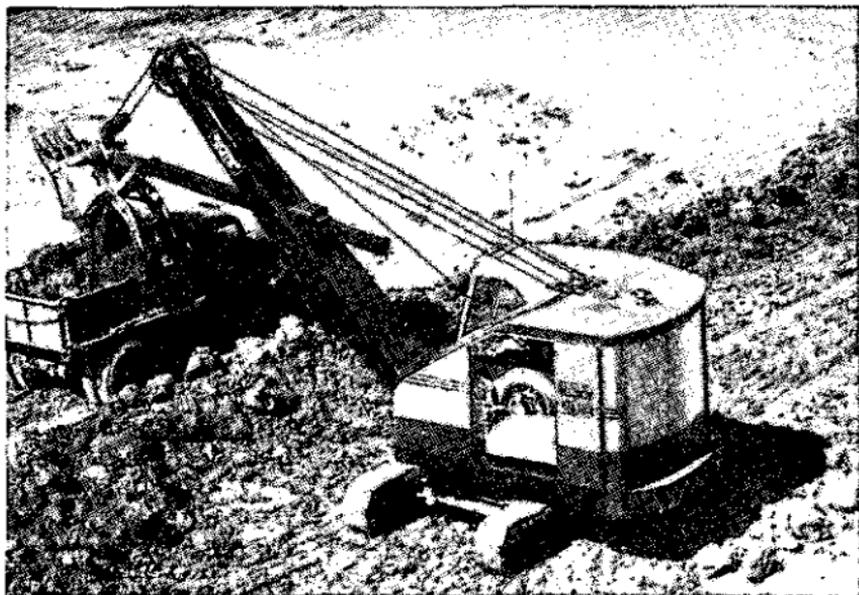
FIGURE 21.—Power shovel loading dump truck.
