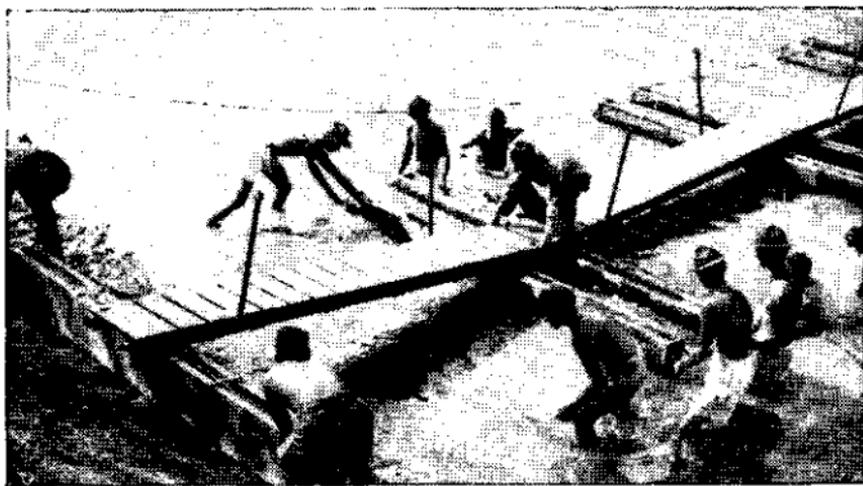
FIGURE 46.—Construction of footbridge by successive bays.
