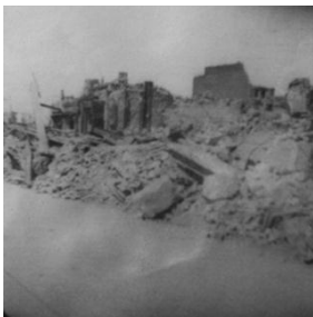
Damage along road
